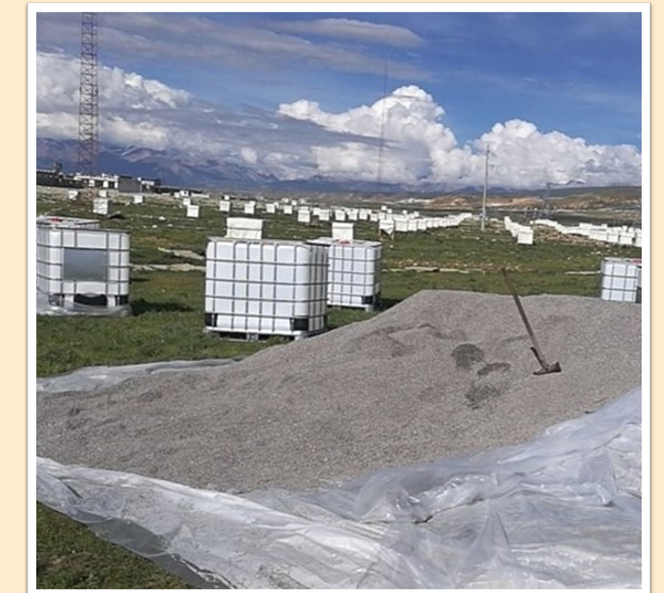
Sand Cube under construction
