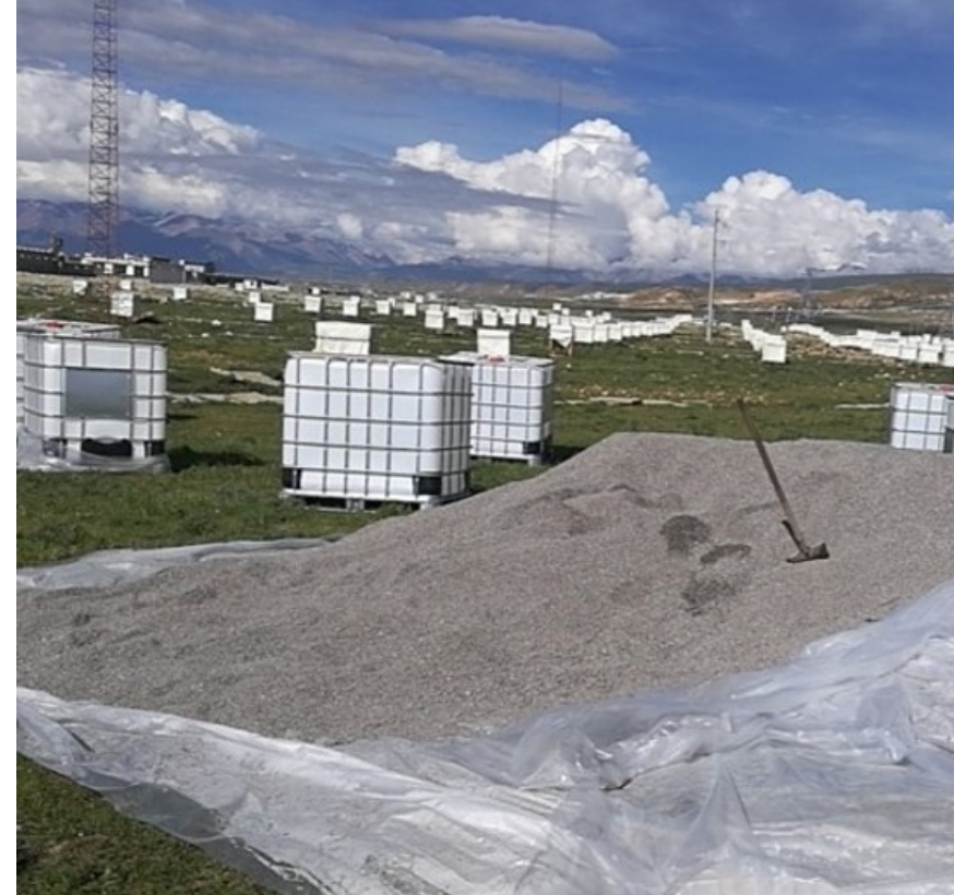
Sand Cube under construction
