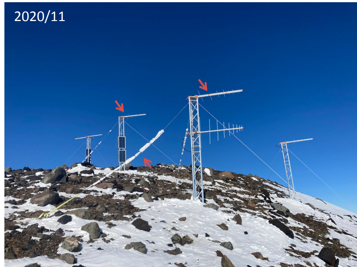
a few guy wires get loose, a few antenna elements damaged
